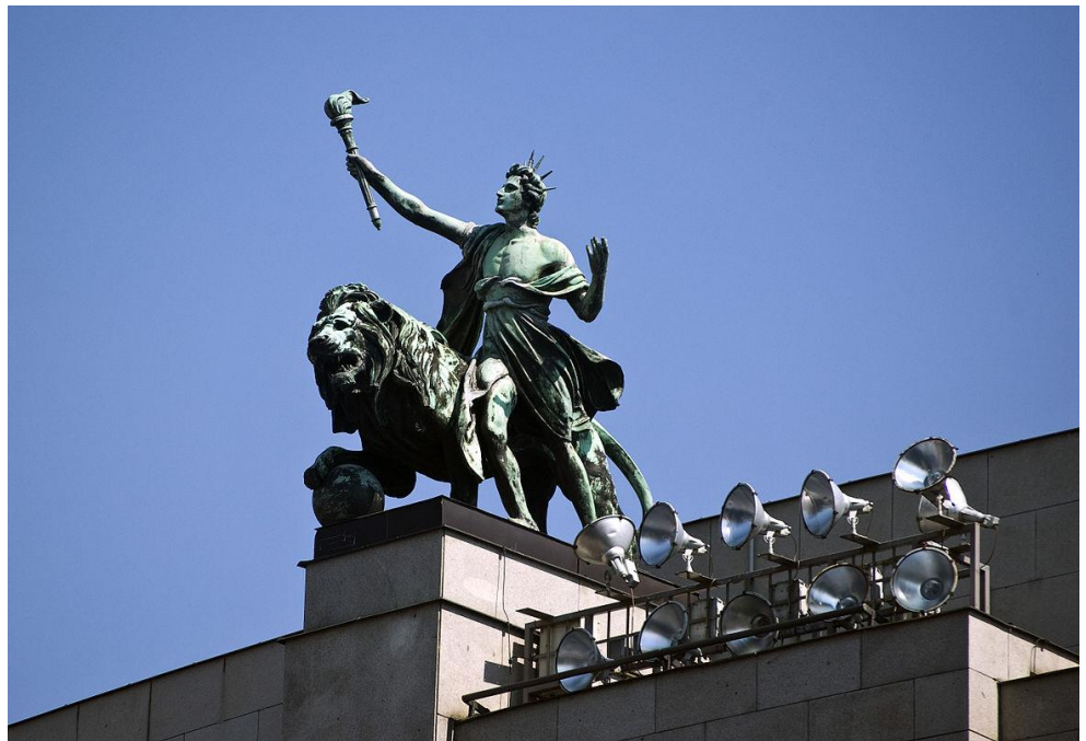
Sculpture on the roof of the headquarters of the Czech National Bank in Prague.
