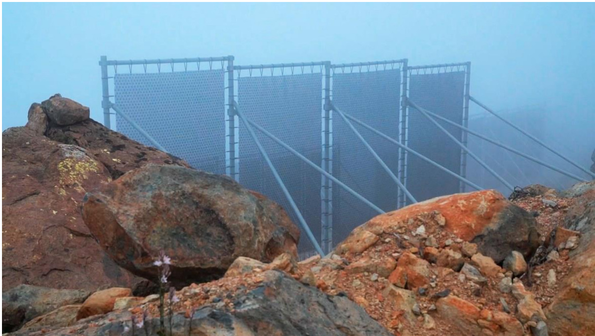
Picture 1. Harvesting fresh water from fog in Ait Baamrane, Morocco
